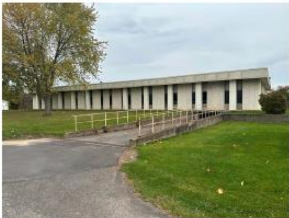
Rear of Building with Access to Basement
