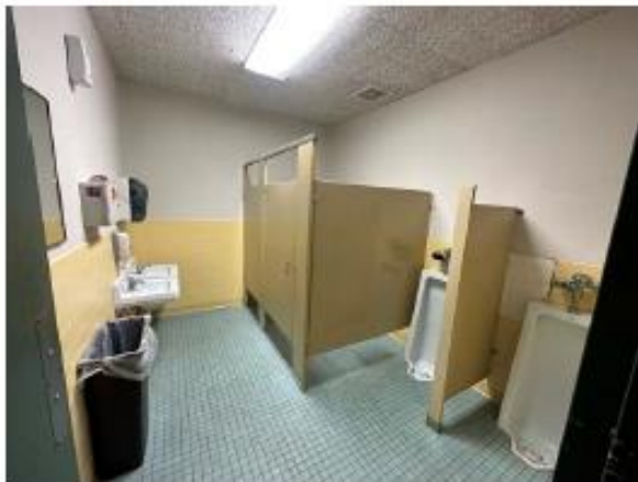
Common Men's Bathroom
