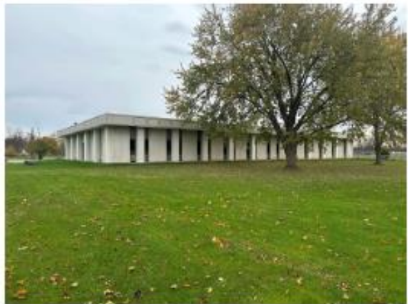
Side/Rear of Building
